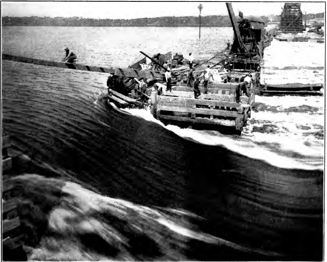
COMPLETING THE LAST SECTION OF THE COFFER-DAM WHICH, AFTER WATER-PROOFING, ENABLED THE CONTRACTORS TO PUMP DRY THE RIVER BED DOWN-STREAM AND SO TO BUILD THE PERMANENT DAM AND POWER HOUSE.
